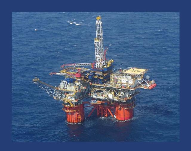
The TITAN is a triple-column deep-draft, floating production facility of a hybrid semisubmersible - spar-type.
